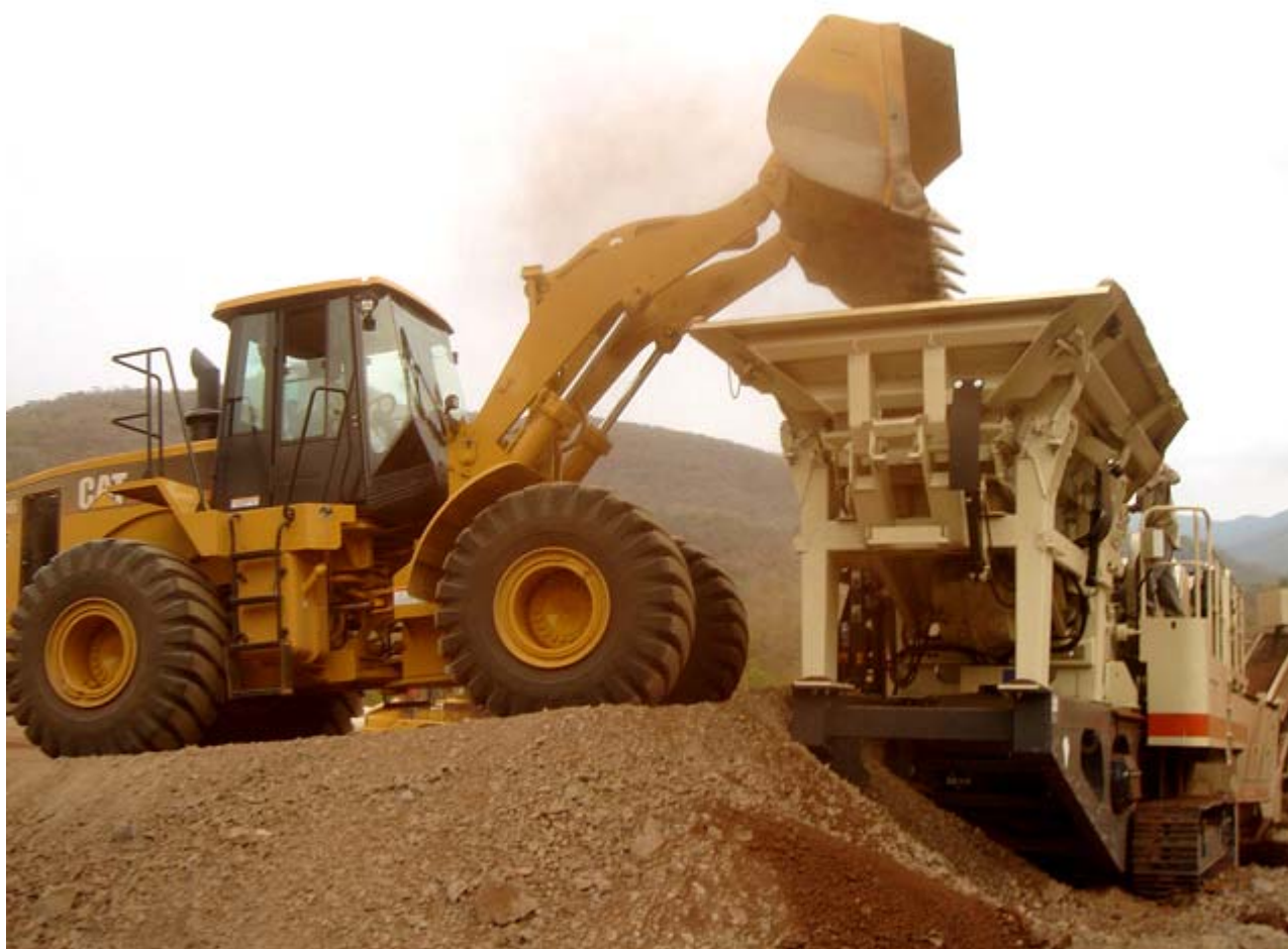
Cat 966G loads Primary crusher at Rio Fox
